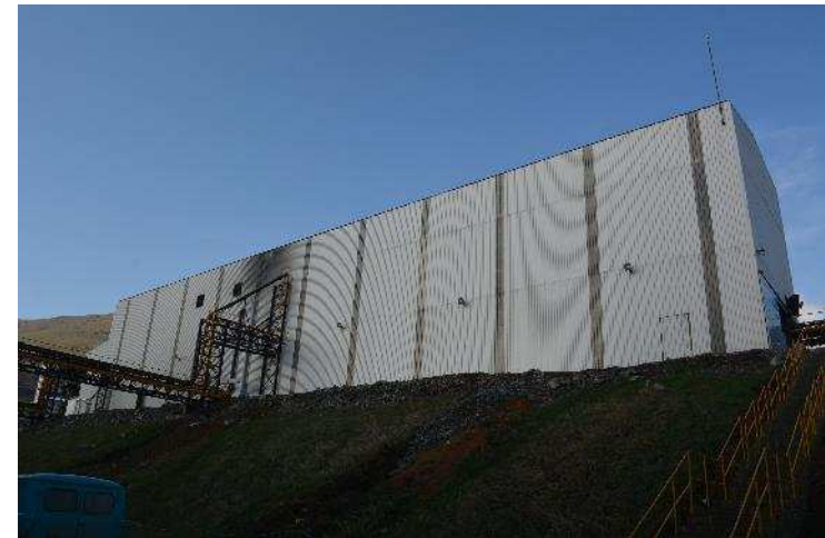
Gedabek - Flotation plant
