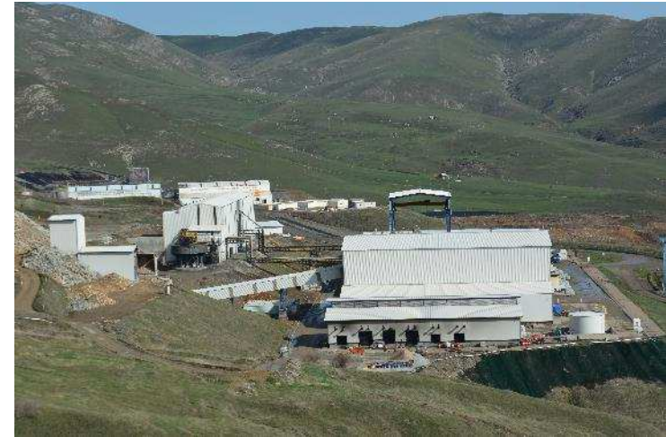
Gedabek - Agitation leaching plant
